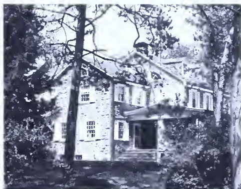
Home eight miles east of Harrisburg in Lower Paxton Township, built of Martinsburg sandstone.
